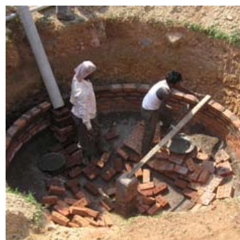
Local masons building a biogas plant (SKG Sangha, India)
